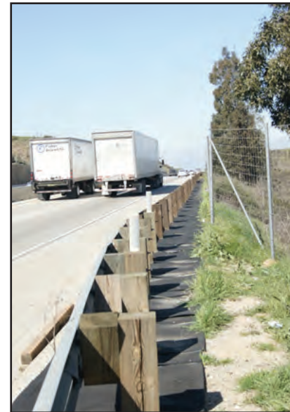
Weed mats installed along Hwy 71.
